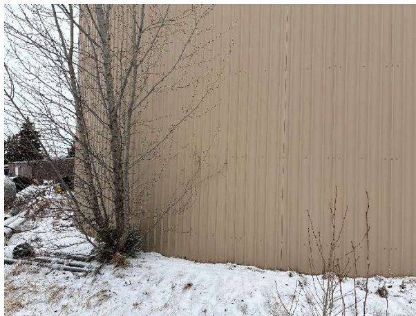
Figure 22: Water Storage Reservoir Wall Cladding
