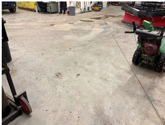
Figure 8: Main WTP Building Slab-on-Grade
