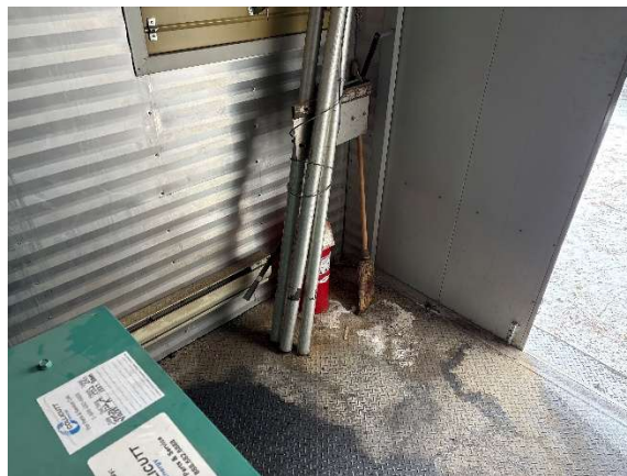
Figure 10: Generator Building Checkered Steel Plate Floor
