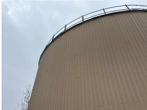
Figure 7: Water Storage Reservoir Walls Exterior
