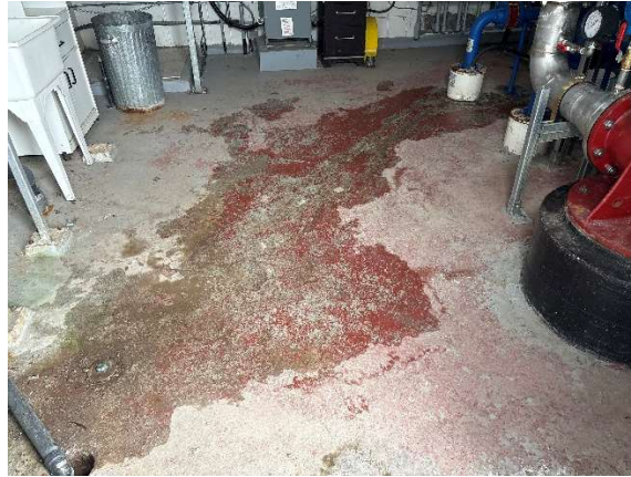
Figure 9: Bulk Water Distribution Building Slab-on-Grade
