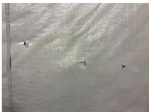
Figure 28: Main WTP Building Plastic Liner Penetrations
