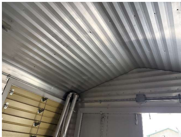
Figure 3: Generator Building Roof Interior
