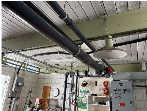
Figure 2: Bulk Water Distribution Building Roof Interior
