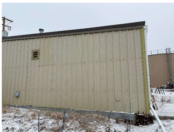
Figure 4: Main WTP Building Walls Exterior
