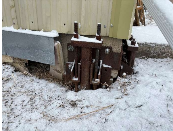
Figure 11: Main WTP Building Southeast Foundation Corner
