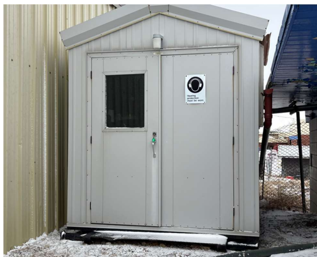
Figure 27: Generator Building Door
