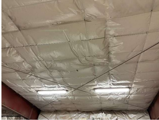
Figure 1: Main WTP Building Roof Interior
