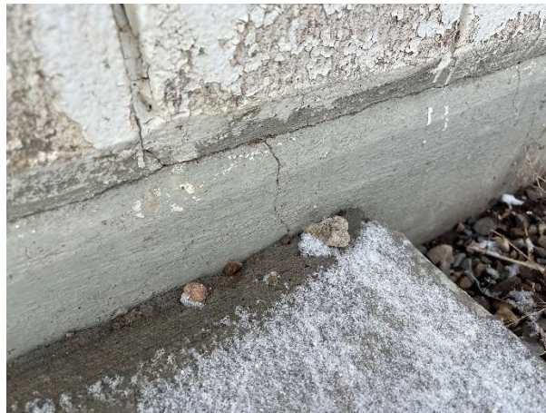
Figure 12: Bulk Water Distribution Building Foundation Wall
