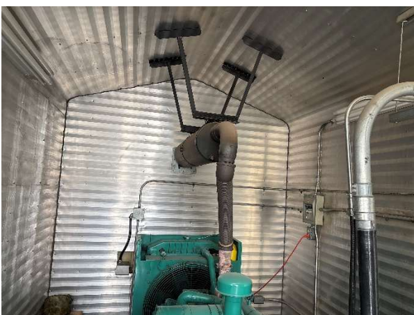
Figure 35: Generator Building Interior Steel Liner
