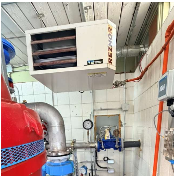
Figure 53: Unit Heater
