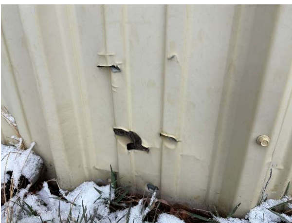
Figure 17: Main WTP Building Cladding Penetrations
