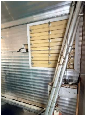
Figure 56: Manual Louver
