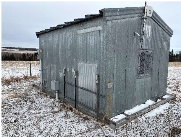
Figure 2: Steel Wall Cladding
