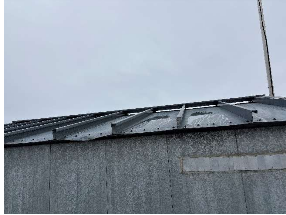
Figure 1: Standing Seam Steel Roofing
