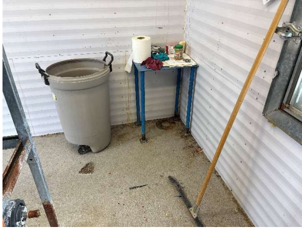
Figure 14: Stained and Ripped Linoleum Flooring
