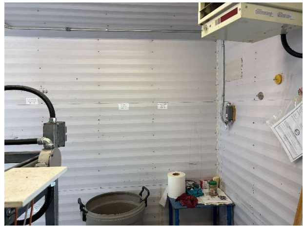
Figure 3: Interior Steel Wall Lining
