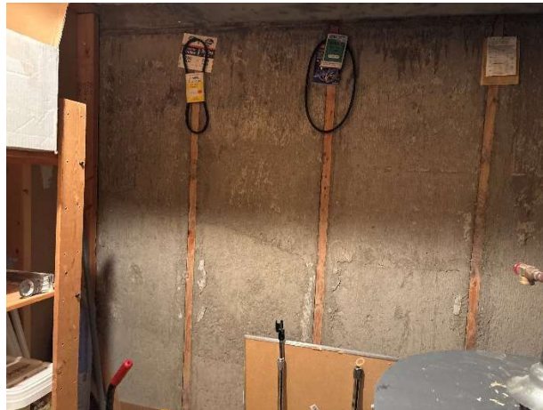
Figure 5: Wood Framing in Concrete Foundation Wall
