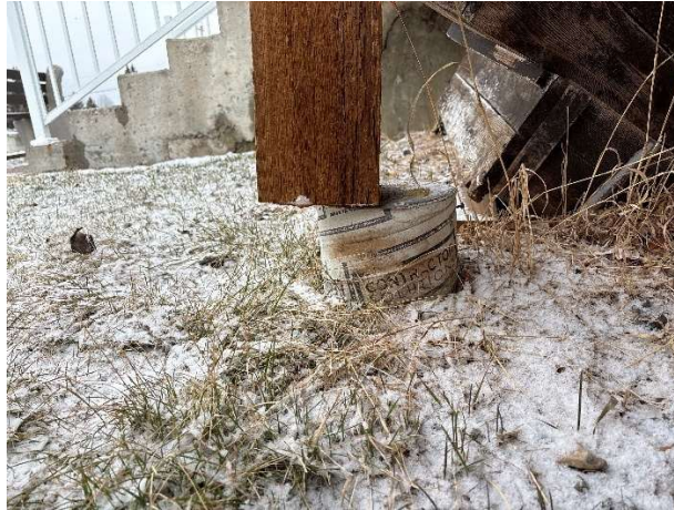
Figure 25: Ramp Post Eccentricity
