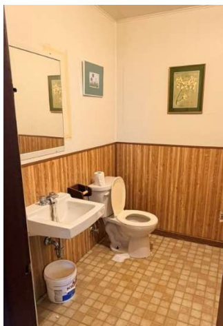
Figure 34: Basement Washroom Fixtures
