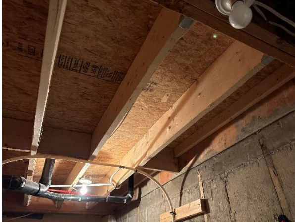
Figure 3: Main Floor Joists
