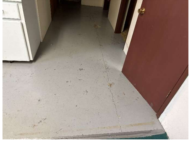
Figure 4: Basement Floor Slab
