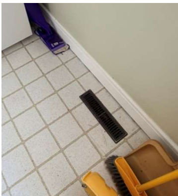
Figure 43: Typical Floor-mounted S/A Double Deflection Grille
