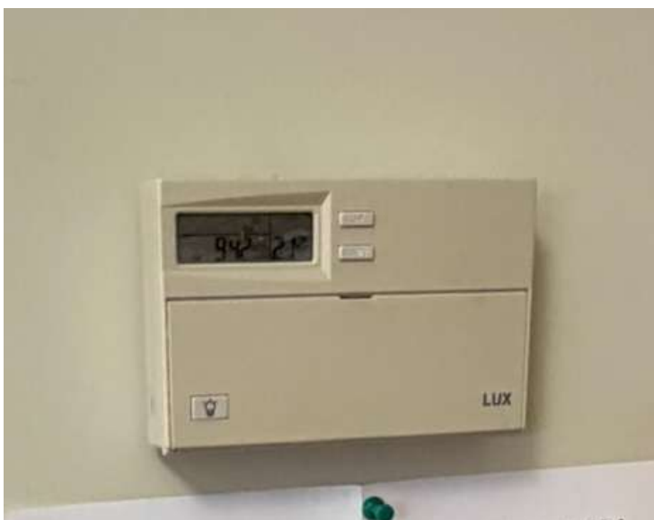
Figure 46: LUX Programmable Thermostat
