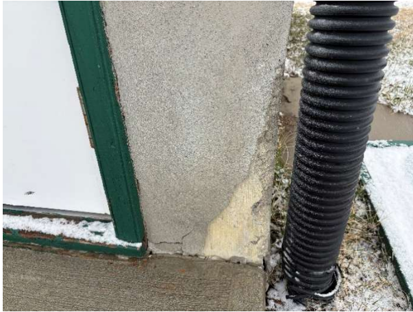
Figure 12: Parging Deterioration
