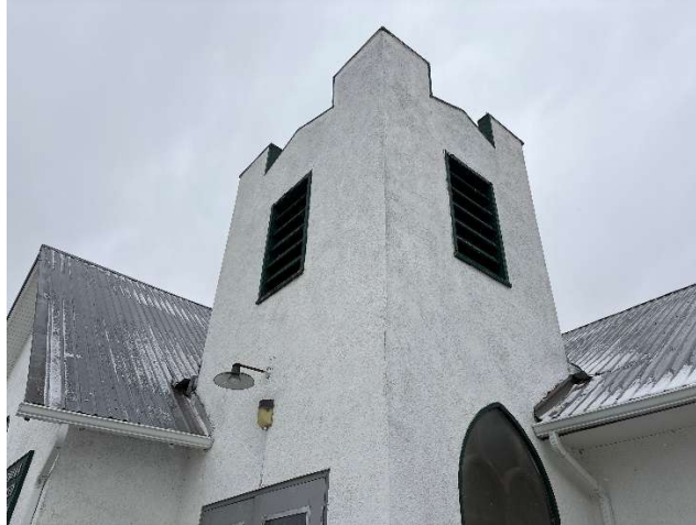
Figure 1: Corrugated Steel Roof Decking
