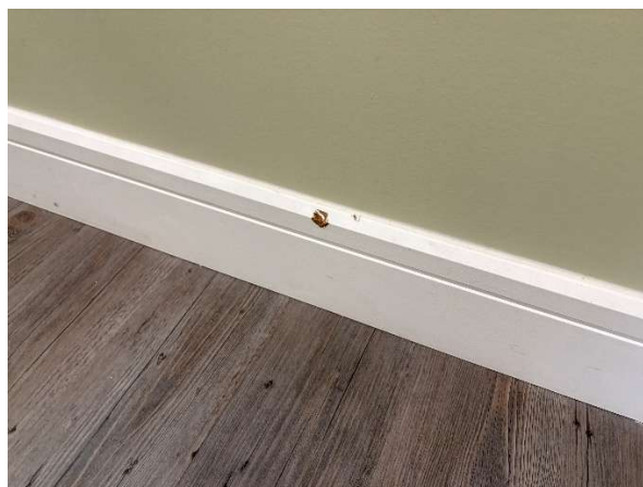
Figure 18: Damaged Baseboard
