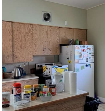
Figure 42: Wall-mounted Exhaust Fan Above Range Cooker
