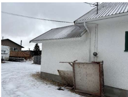
Figure 8: Missing Eavestrough
